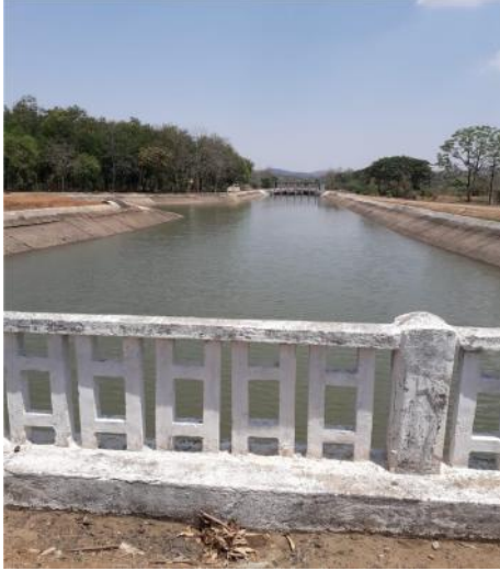
Tawa Main Canal
