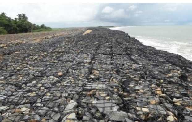
Geo tube installation to control soil erosion in Pentha, Odisha
