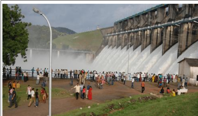
Panoramic View of the Tawa Dam
